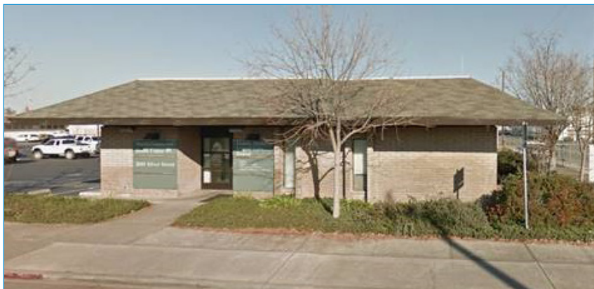
Photograph of SCHC former health center facility in Anderson, CA.
