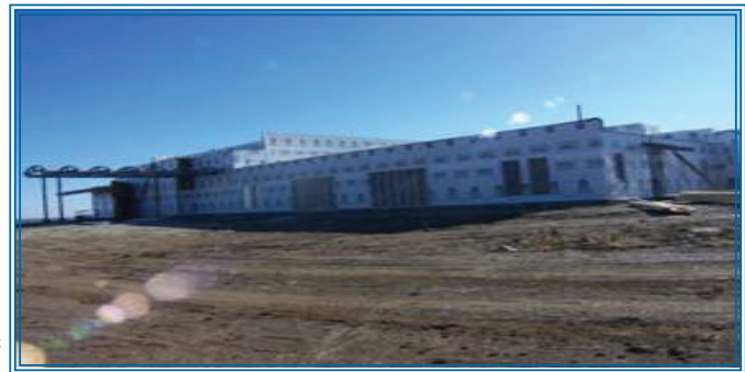
Construction progress to date
